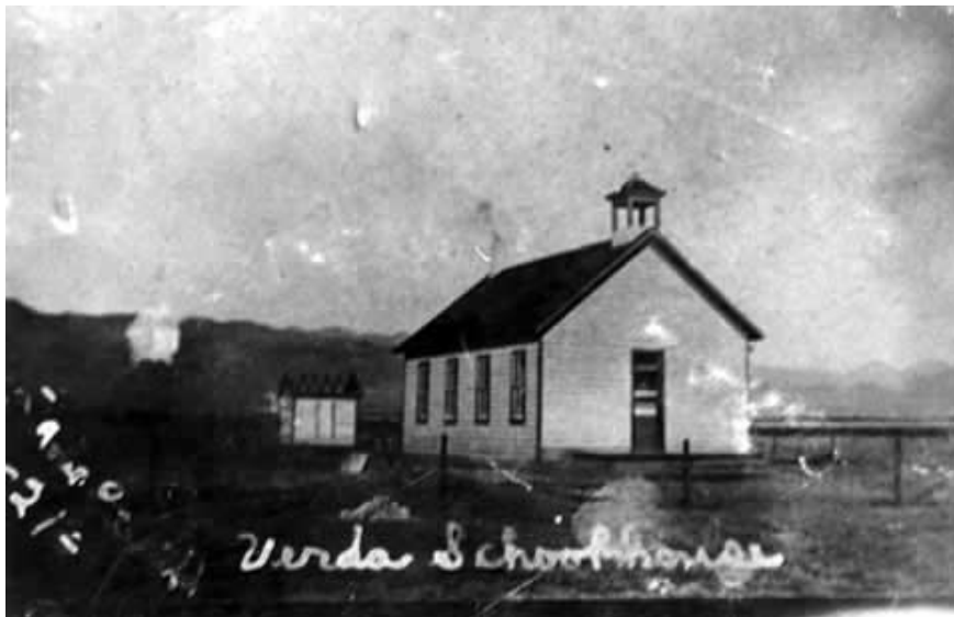
Photograph 6. A schoolhouse was built in Verda (circa 1912) to serve the needs of the residents in the southern end of the project.
