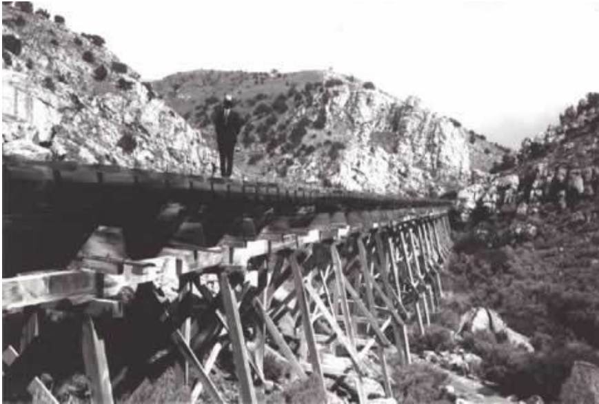
Photograph 4. An impressive flume was built down Goshen Canyon, sections of which were supported on a wooden trestle. Circa 1910.
