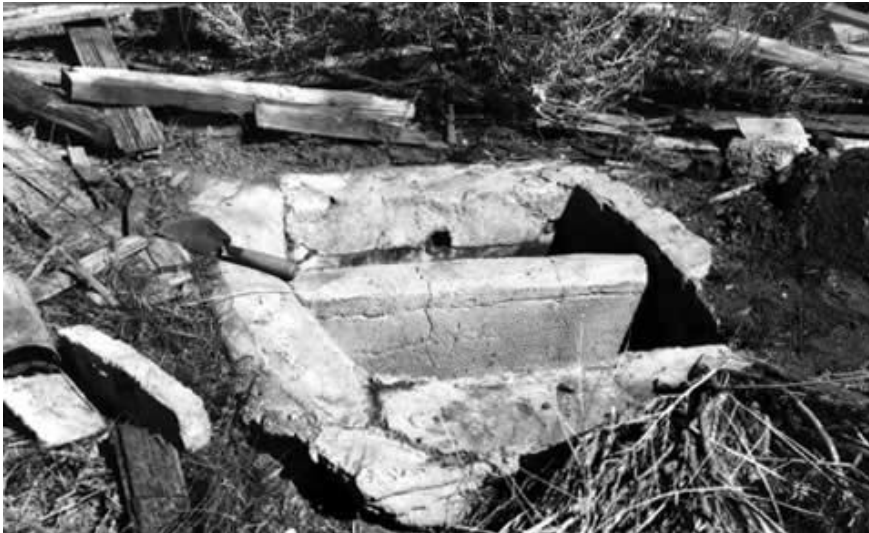
Photograph 10. Before water entered the cistern it was filtered in a small concrete box which contained sand and charcoal. Circa 1984.
